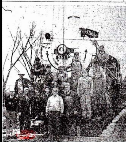
THE END OF A LONG, LONG JOURNEY for "Old 561," Union Pacific's gift to the city of Columbus was completed when the crew shown above moved the 51-year-old engine onto its permanent site in Pawnee Park. The accomplishment was completed in less than three days by a crew of retired railroad men, active railroaders and the city park crew under the supervision of Jake Gluz of the park board. Shown in the photo from left to right bottom row are: Nels Nelson, park commission; Frank Kosiba, railroad; John Forney, railroad; Jake Gluz, park commission; Perry Loveless, railroad. Second row, left to right: Rudy Skoll, park commission; Bill Trotholz, park commission; Mike Mimick, railroad; Henry Pensick, railroad; Fred Mathes, park commission; Leonard Ferguson, park commission; William Semrau, railroad. Top row left to right: Clarence Pensick, park commission; John Novicki, railroad; L. E. Shilling, railroad; Ed Kudron, caterpillar operator. Walter Regl of the park commission and Charles G. Bittner of the railroad were also members of the crew but were unable to be present for
